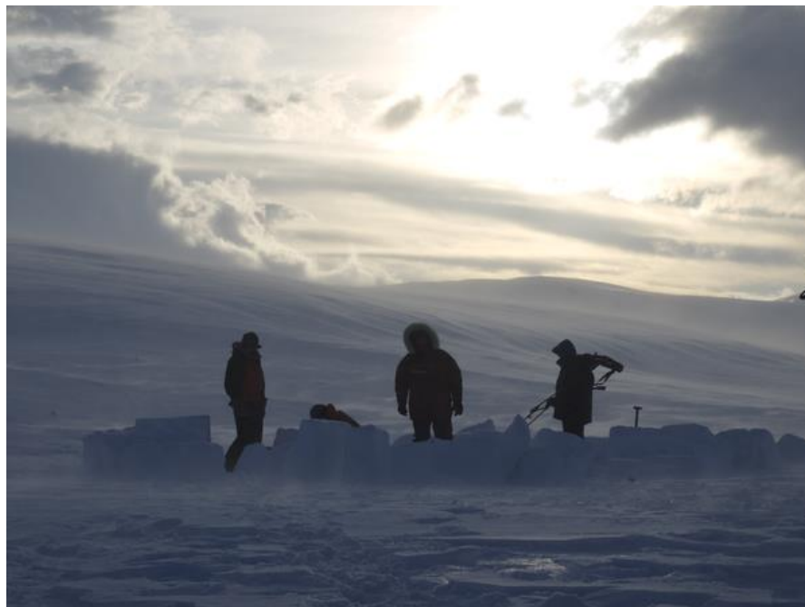
Process of building an igloo with snowbrick method in mid-way
